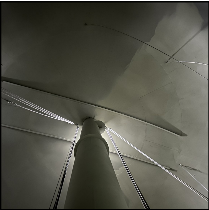
Prime coat of Tnemec Series 91H2O
