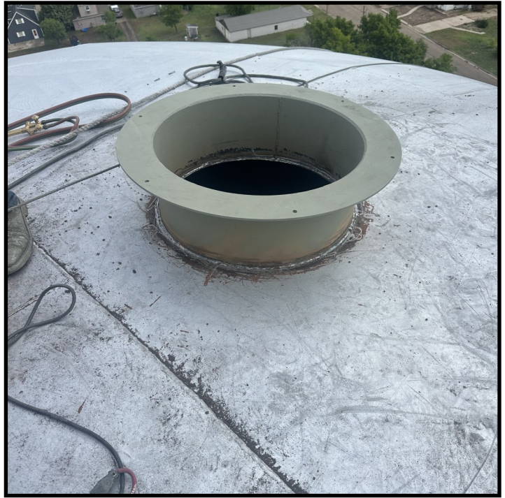
Flange installed for new vent
