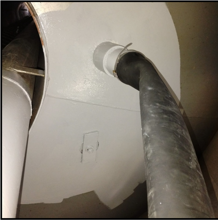
New flexible piping installed at bottom of bowl
