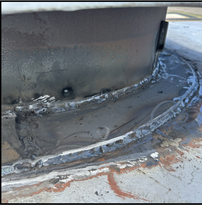
Sealing of floating dry riser
