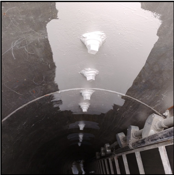
Example of interior dry touch-up
