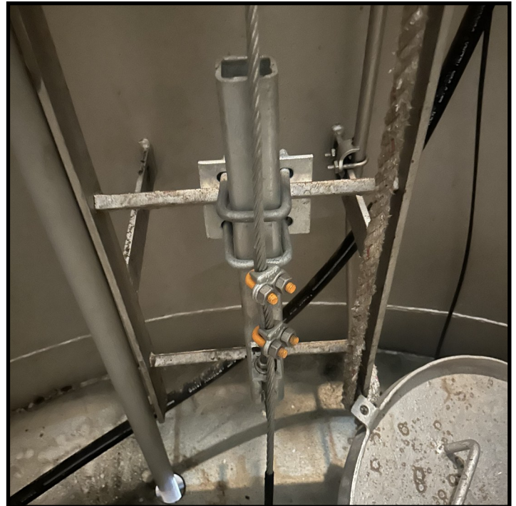
Cable safety climb devices installed at all interior dry ladders
