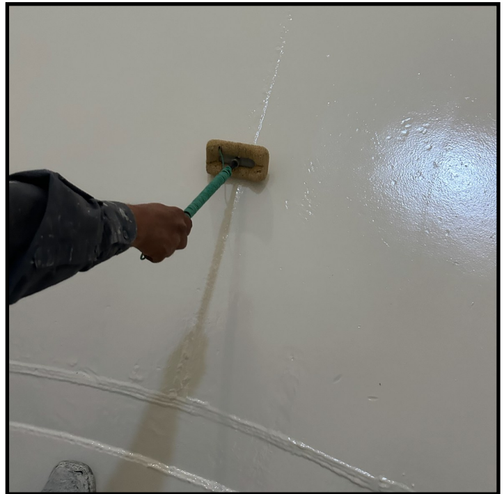
Tank interior holiday detection performed prior to disinfection
