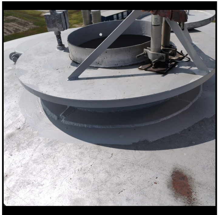
Sealed roof access/riser
