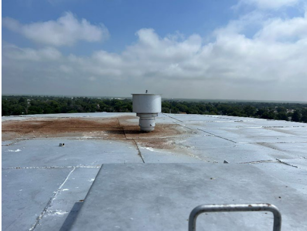
Exterior Center from ladder
