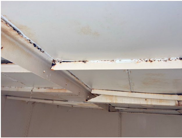
Interior Roof and Support Structure
