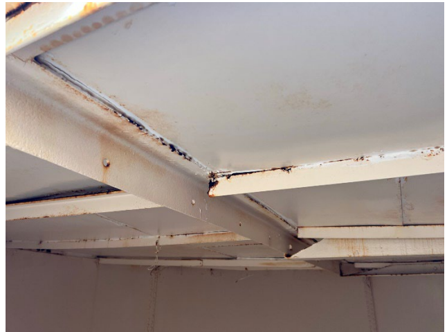
Interior Roof and Support Structure
