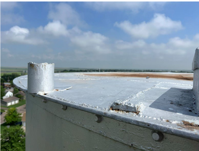
Exterior Angle Roof to Sidewall
