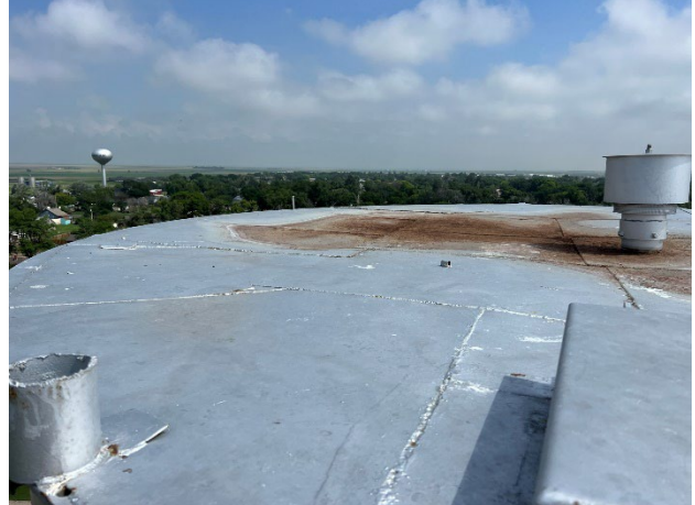
Exterior Left from ladder
