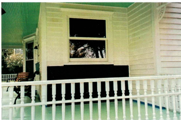
2004, a new window replaces the east front door on the front porch, bringing this area back to original design. Installation by Curtis Hurd and summer crew.
