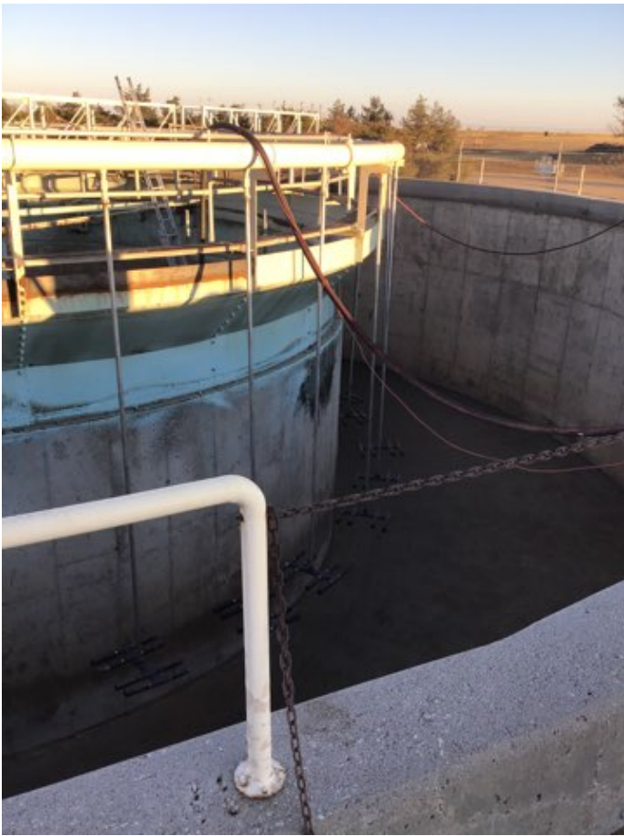
Photo Description: Clarifier before surface preparation.
