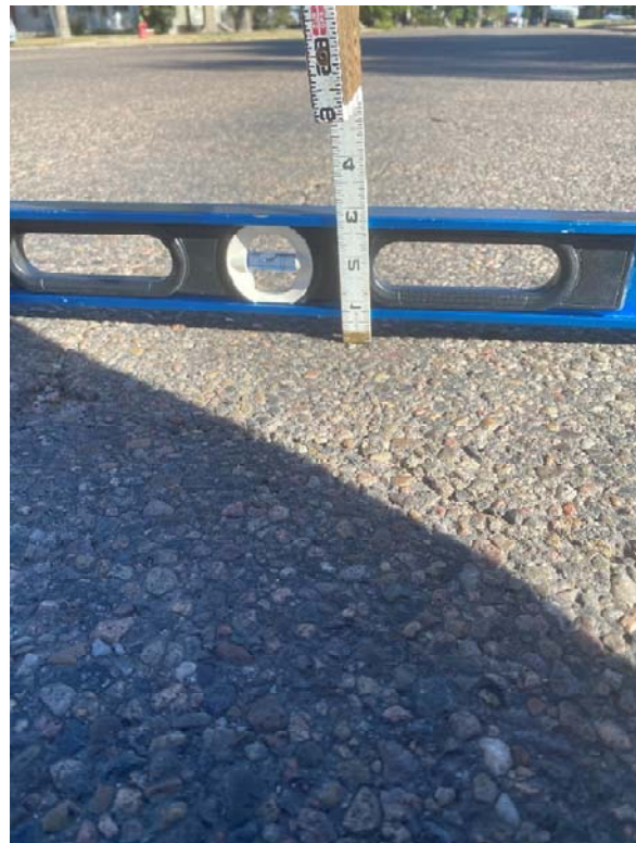
Typical Rutting found Throughout Project
