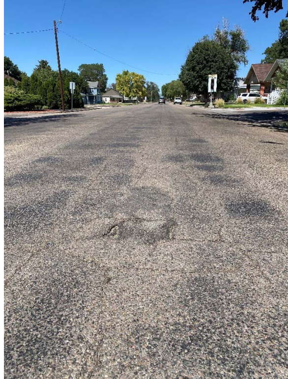
Looking North – Typical Block Cracking
