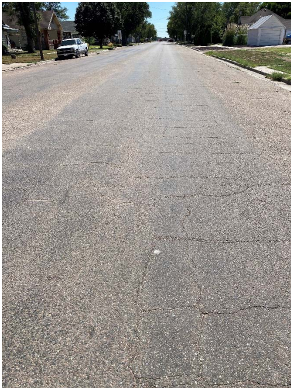
Looking South – Typical Block Cracking
