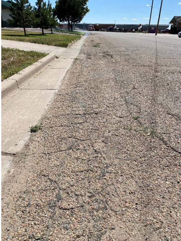
Typical Alligator Cracking and Failure at Curb
